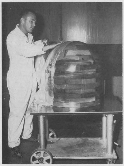
FABRICATION of dust cover for an outdoor camera is started here by Richard Olive. He is placing a layer of resin-impregnated glass cloth on a wood mold. He will build the layer to  $\frac{1}{2}$ s" thickness.
